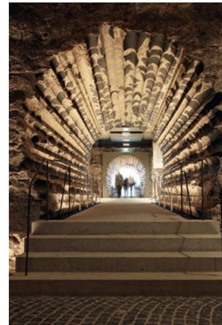
Ill. 2 Passageway through the foundations of the south tower in the new entrance building on the cathedral's south side
